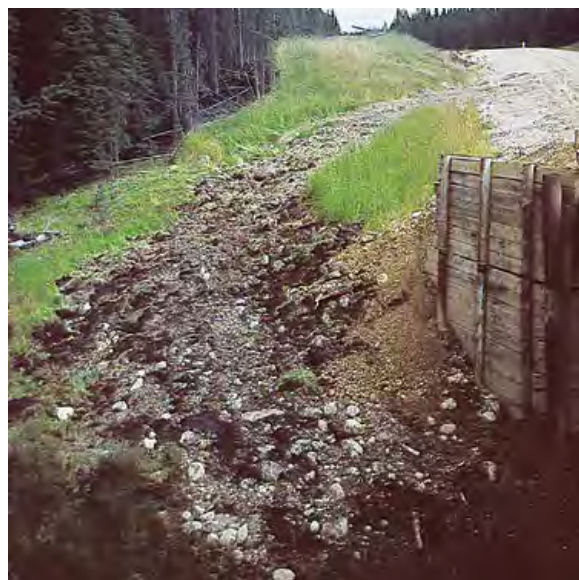
Keep road drainage under control. Even with grass cover, runoff and sediment have flowed around this abutment and drained directly into the stream.
