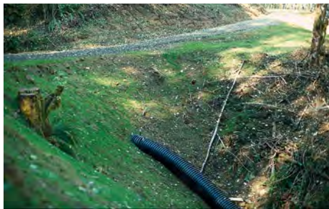
The flexibility of a plastic pipe makes it a popular alternative to a metal culvert.
