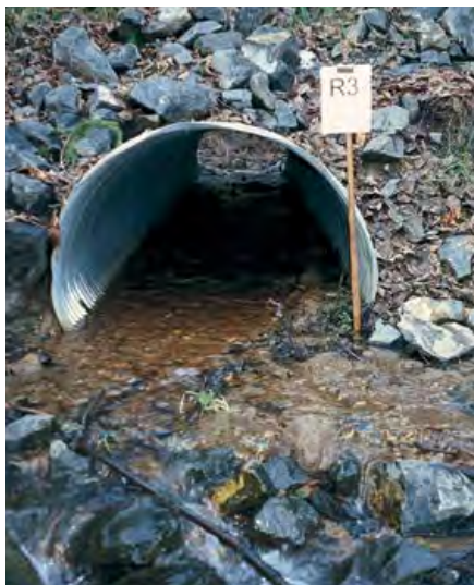
Round, galvanized corrugated metal pipe sunk into the streambed to allow for fish passage.
