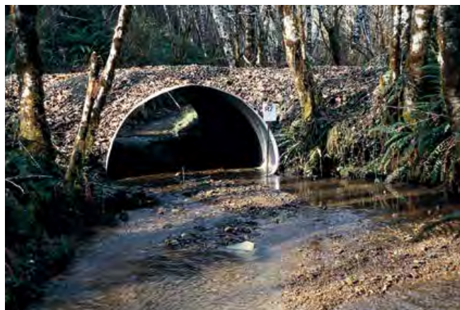
Arch culvert on a low clearance road, sunk into the streambed to allow for fish passage.
