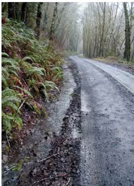
Durable rock surface on a log hauling road during heavy rain. Notice that the water in the ditch is clean.
