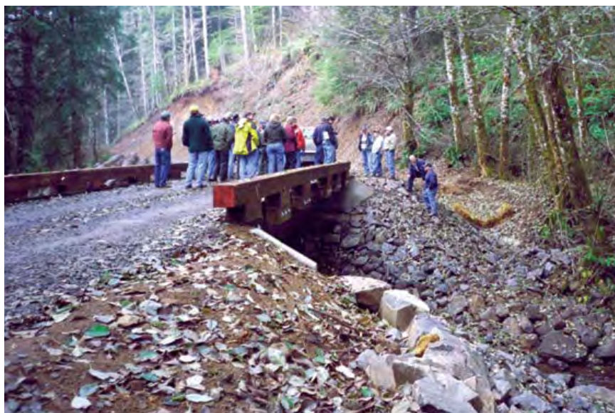
Bridges are best for large streams and those plagued with floatable debris problems. Bridges and bottomless arch culverts have the least impact on fish when installed properly.
