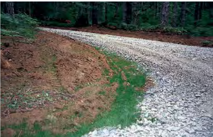
Road surfacing can double the cost of a road. However, gravel roads can provide all-weather access, reduce road maintenance costs and protect water quality by covering the soil with a weather-resistant surface.
