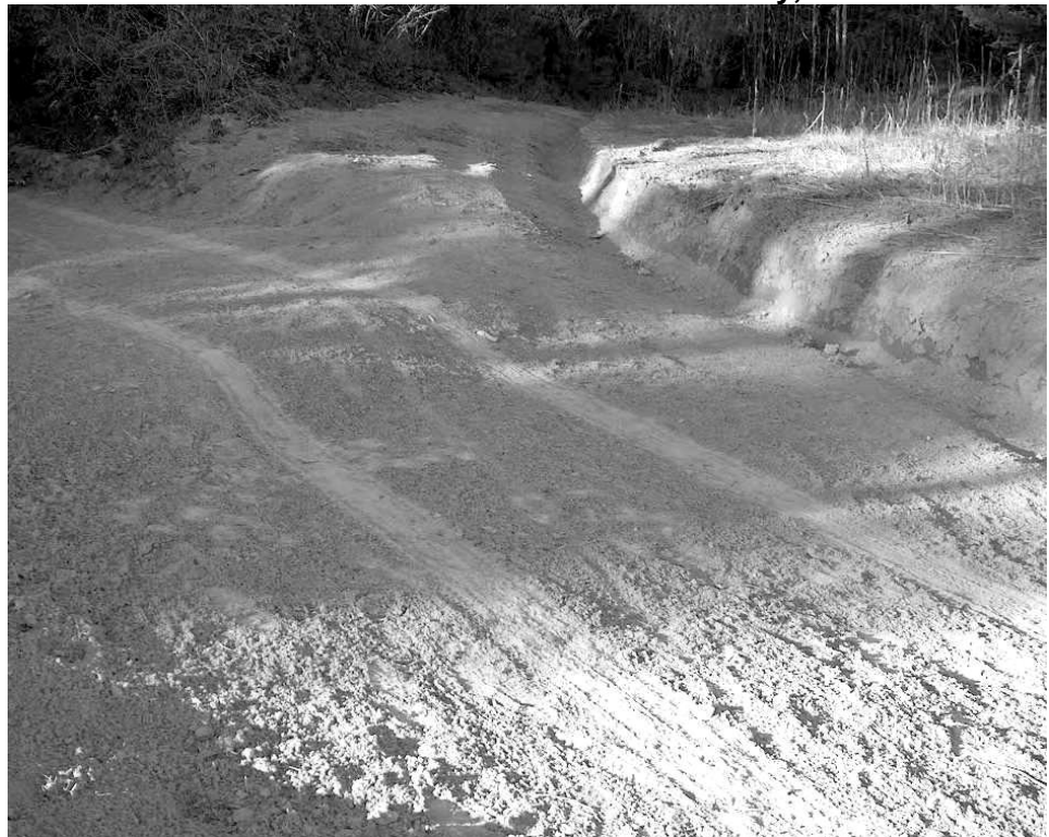
Figure 5F: A turnout, used as a wing ditch alongside a forest access road in Henderson County, N.C.
