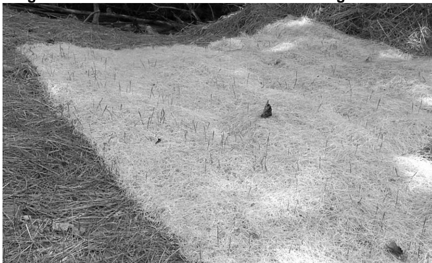
Figure 11D: Erosion control mat installed for groundcover
